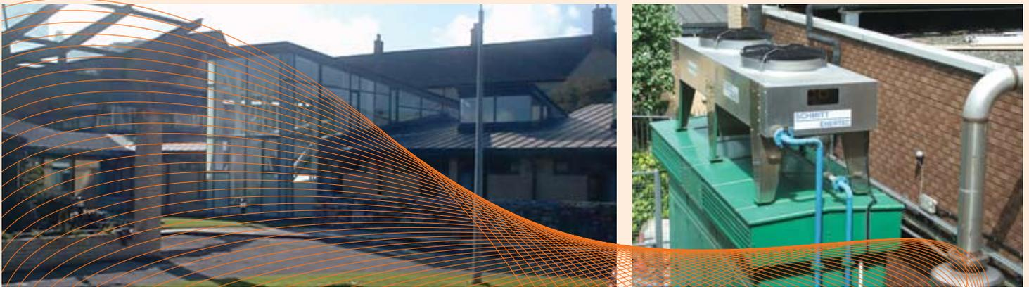
**Technology:** 334 kW<sub>e</sub> and 497 kW<sub>th</sub> reciprocating gas engine CHP to provide heat, electricity and hot water to Saint Patrick's Hospital
